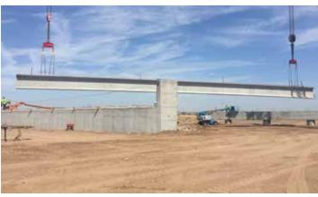
Placing a 174-foot girder, the longest precast concrete girder in Arizona
