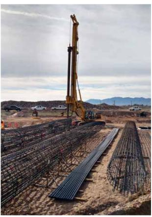
Drilling shafts and installing rebar (ADOT Photo)
