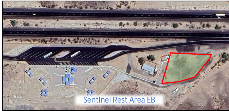
Figure 2-4. Sentinel Overflow Parking
