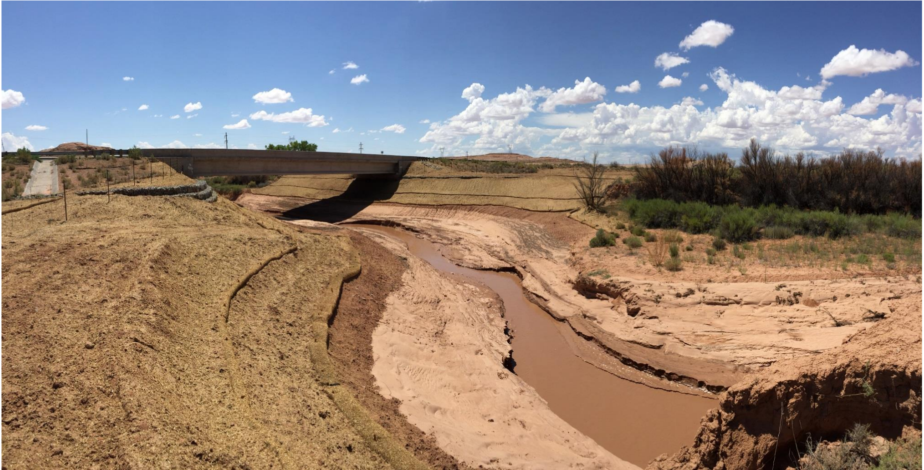
November 2017 – State Route 160 Laguna Creek Bridge (Final grading and seeding)
