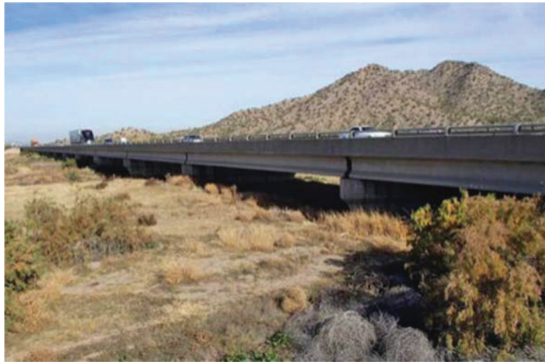
Figure 32. San Pedro Bridge over the Gila River, SR-80, Arizona.
