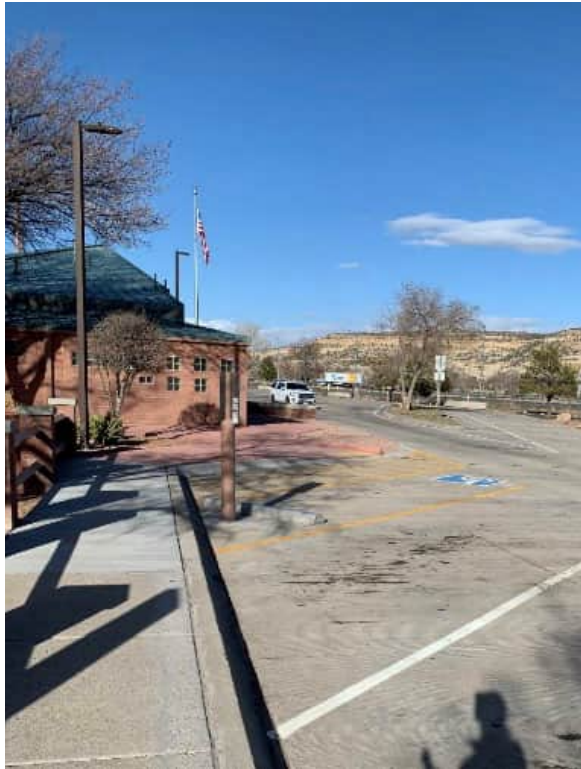
Figure 4-5. ADA Improvements at Rest Areas
