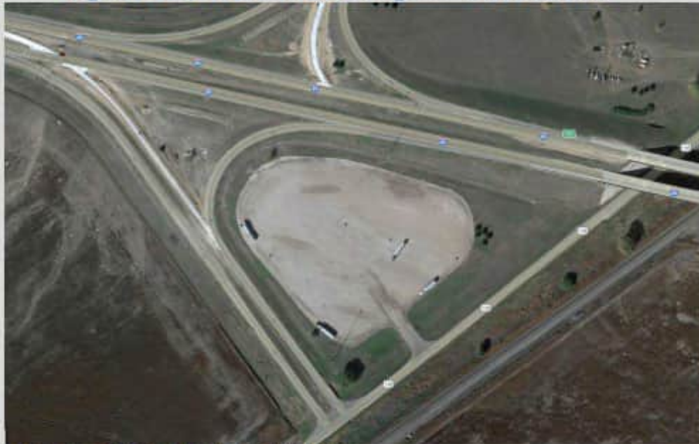
Figure 2-12: Low Cost Truck Parking Solution in Nebraska
