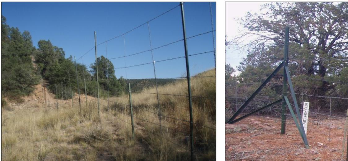
*Figure 2.* Application of retrofitted ROW fencing using 10-foot T-posts and barbed wire to extend the fence to 7.5–8 feet, with a metal in-line support posts for strength (left). Existing ROW fence corner braces were raised and supported with new angle braces bolted to the upright and bedded in concrete (right). Fencing retrofitted on State Route 260.
