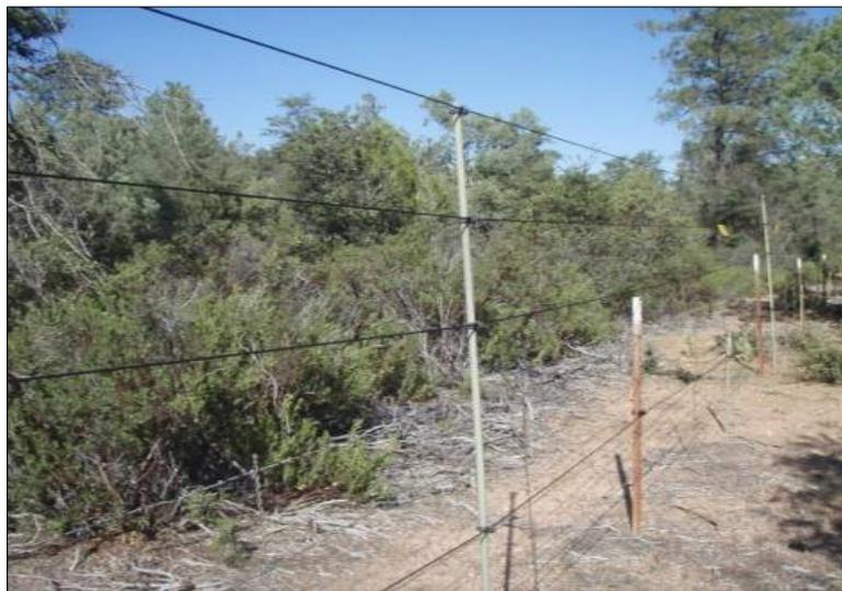
*Figure 4.* Application of modified ROW fence raised to 8 feet with ElectroBraid™ braided rope electric fence and fiberglass posts, with an electrified “kicker” mounted on the outside of ROW fence T-posts. Fencing retrofitted on State Route 260.
