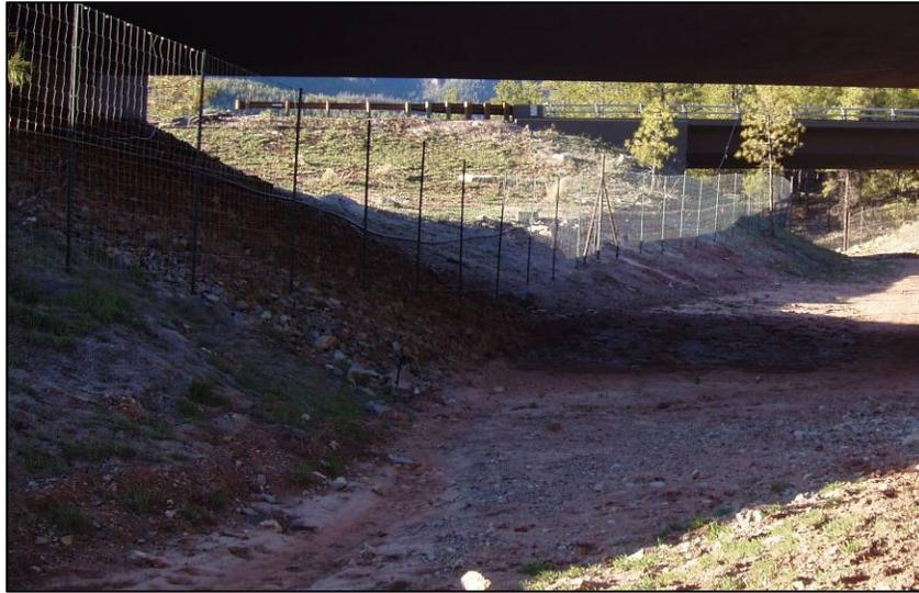
*Figure 1.* Standard 8-foot wildlife fence erected at a wildlife underpass along State Route 260. Note the woven wire, T-posts space 20 feet apart and metal support posts.
