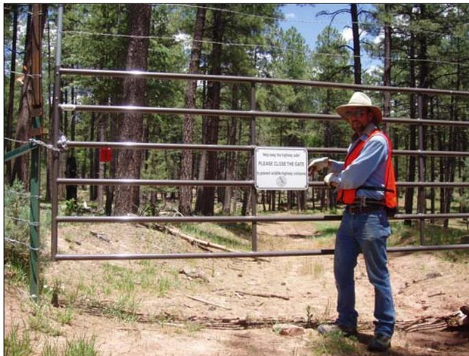
*Figure 6.* Modified 6-foot Powder River gate installed on a lateral access along State Route 260. Gate was raised to 8 feet with a barbed-wire stinger above the top rail to preclude animals from entering the fenced ROW. Note the sign imploring users to close the gate.
