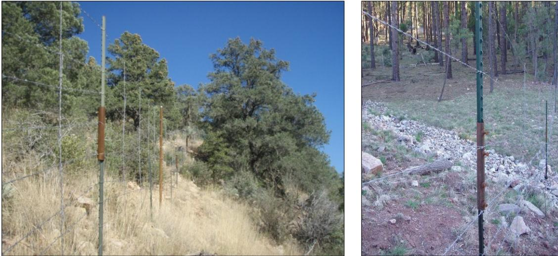
*Figure 3.* Application of retrofitted ROW fencing using T-post sleeve extensions and barbed wire to extend the fence to 7.5–8 feet, with a metal in-line support post for strength (left). Close-up of the T-post sleeve extending the existing T-post upward with bolts securing T-posts in place (right). Fencing retrofitted on State Route 260.
