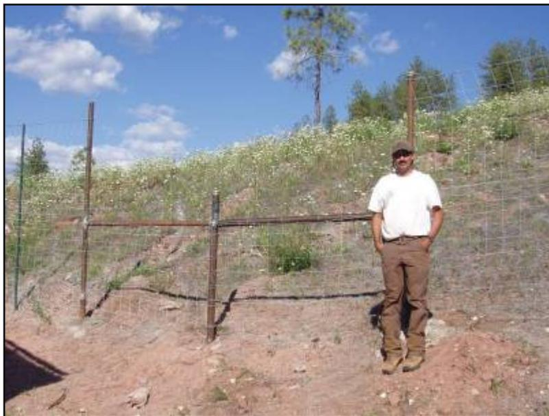
*Figure 4.* Wildlife slope jump located along State Route 260, where animals jump from over the lowered section of fence to escape from the fenced corridor (uphill side). The slope deters animals from jumping over the fence and breaching the fenced corridor.
