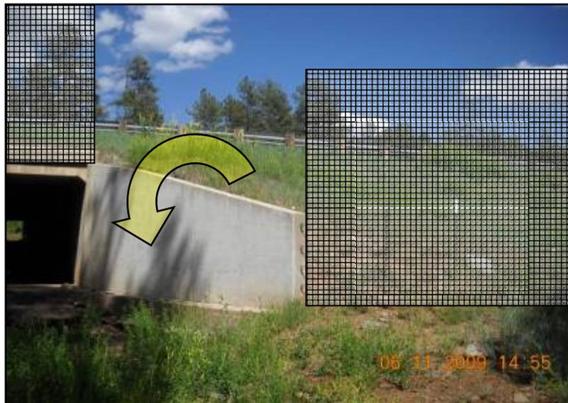
*Figure 5.* Box culvert headwall that is conducive to being retrofit to function as an escape jump, with raised fencing being erected on each side of the headwall, allowing animals to jump off the top of the headwall to escape the fenced corridor.
