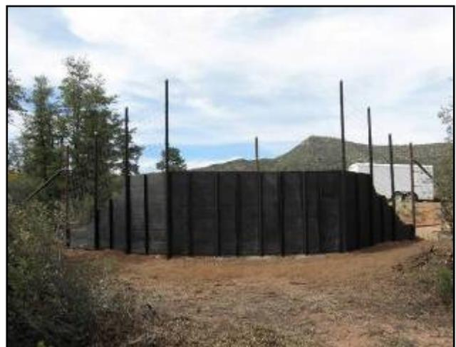
*Figure 3.* Scaled-down ramp constructed along the Preacher Canyon section of State Route 260; the retaining wall for this ramp was constructed from recycled plastic planks.
