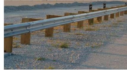
**MGS SOIL BACKING:** Standard guidance for installation of guardrail (MGS and G4) is a minimum 10H:1V into the face of the rail, and 2 ft. minimum of 10H:1V behind the post, which is also the ADOT proposed requirement. When this is not practical to provide, the MGS has been successfully crash-tested to MASH with the standard 6' post placed right at the slope break point. (Reference: FHWA letter B-211, dated 06/10/11).
