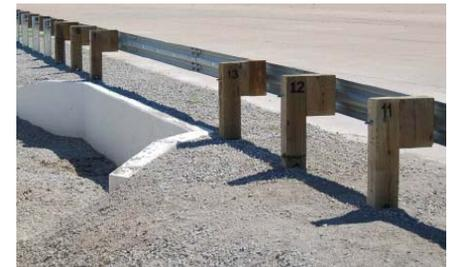
**MGS TRANSITION DESIGN:** The MGS system is compatible with most existing Thrie-beam to rigid barrier/bridge railing transition designs with the use of a non-symmetrical W-beam to Thrie beam 10-gauge transition section and a modified post layout upstream of the Thrie-beam. Steel or wood posts can be used. The recommended design was successfully crash-tested under MASH criteria (References: FHWA letters B-231, dated 01/27/12 and B-236, dated 05/30/12).
