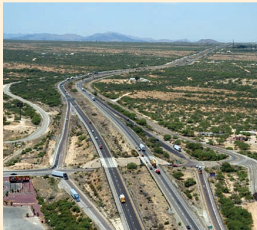
Aerial view of the I-10/State Route 90 Traffic Interchange.
