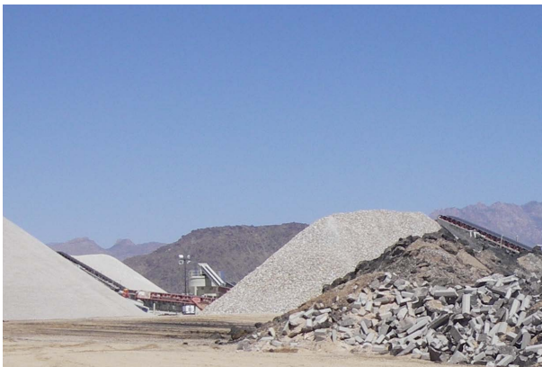
Figure 9.4 Batch plant and crusher.
