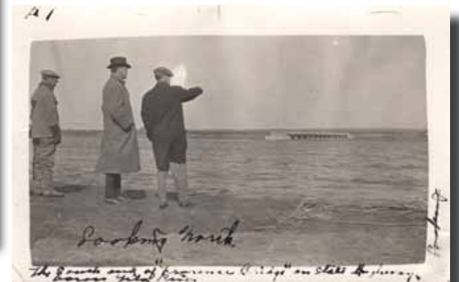
Three men viewing Gila River from bank at Florence, Arizona, during 1916 flood. They are at looking north toward a portion of the bridge isolated in the river.
