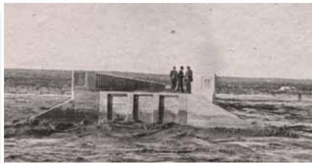
A group of men stand on the bridge after the Gila River destroyed bridge approaches during 1916 flood.
