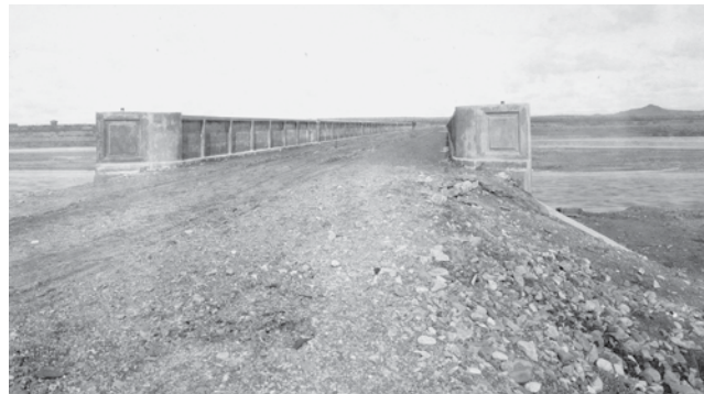
This is the bridge designed by Territorial Engineer James B. Girard and built in 1910. It’s the bridge involved in Federal Aid Project No. 1 in 1917.
