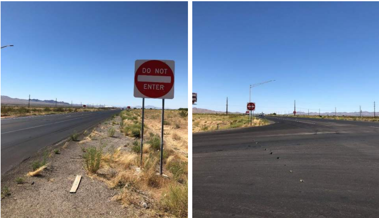
Left – US 93 SB viewing north from the median crossing.
