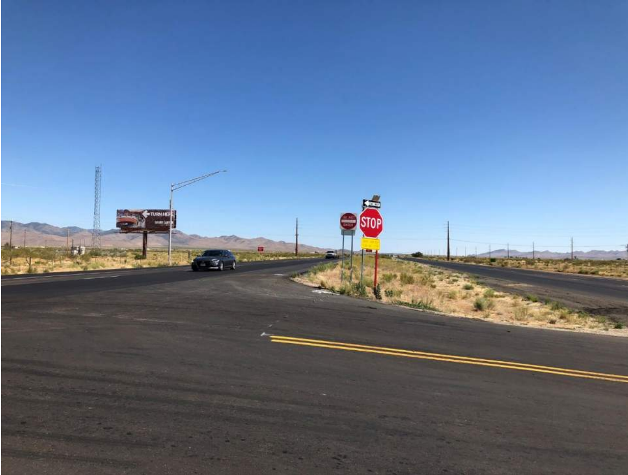
Viewing south from north of median crossing
