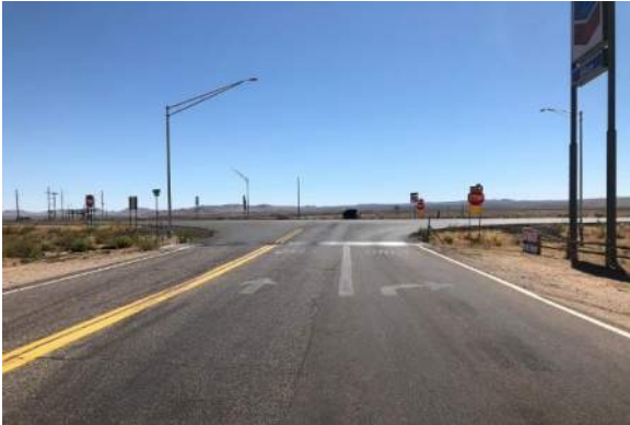
Pierce Ferry Road viewing west
