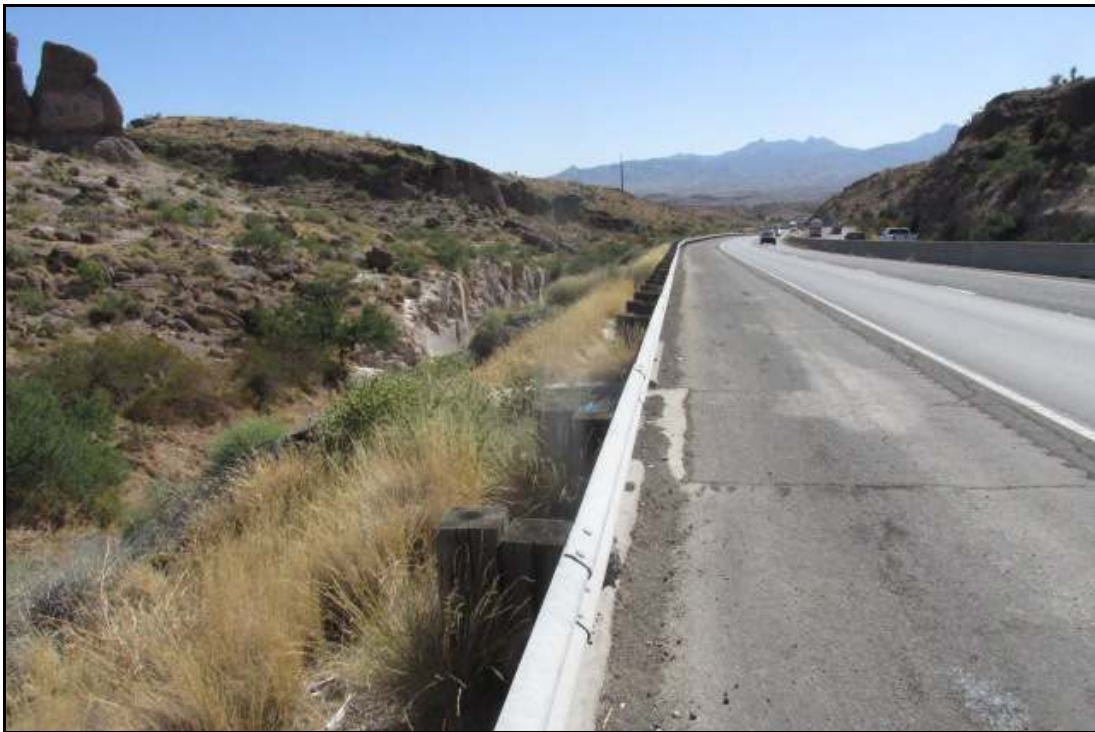
Photograph 8. View west from US Highway (US 93) near MP 69.5, the eastern project limit. Photograph date: October 2, 2019.
