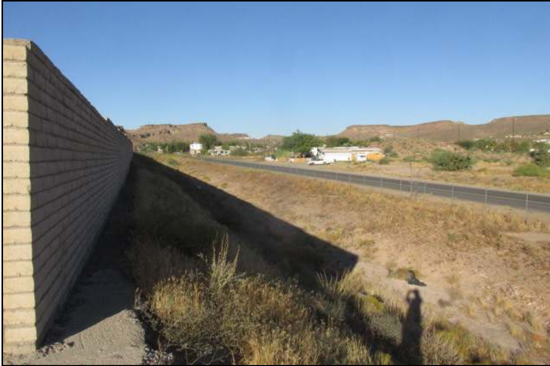
Photograph 13. View southwest of the I-40 north side drainage channel near MP 51.4. Photograph date: October 2, 2019.
