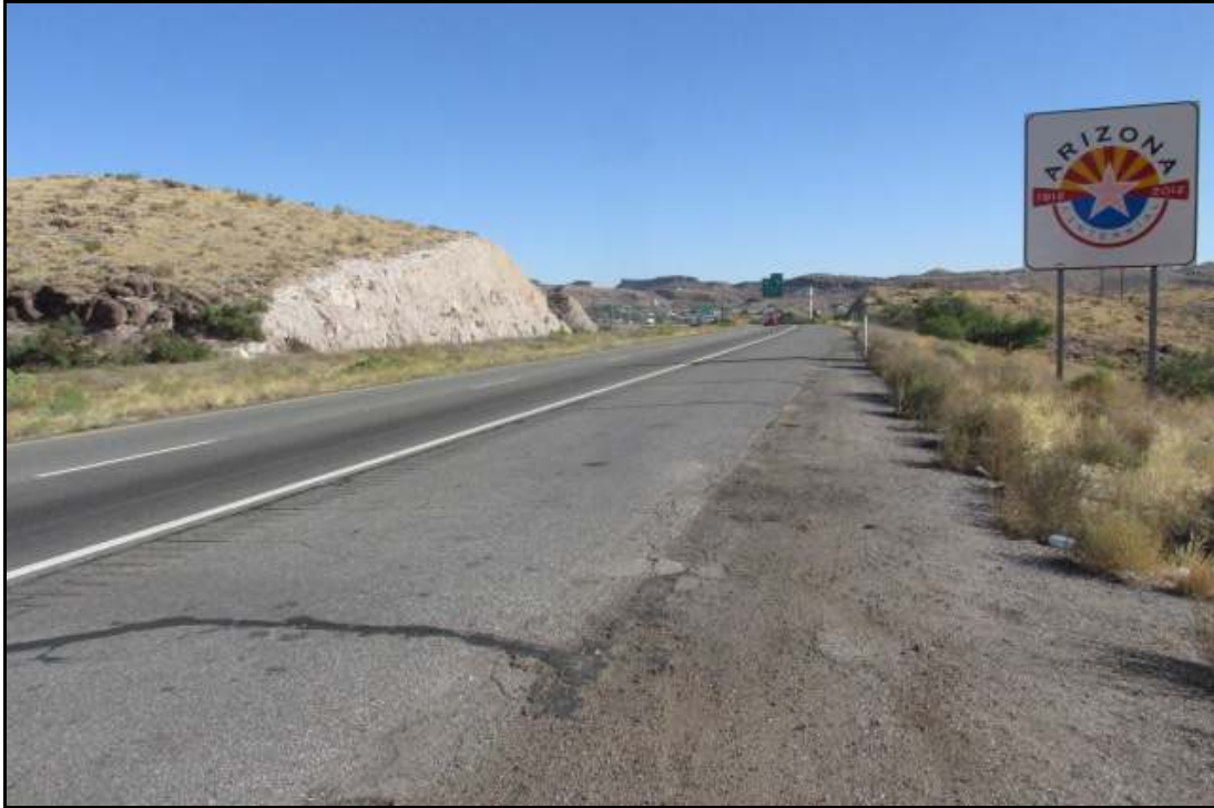
Photograph 1. View northeast from Interstate 40 (I-40) near milepost (MP) 48.3, the I-40 southern project limit.
