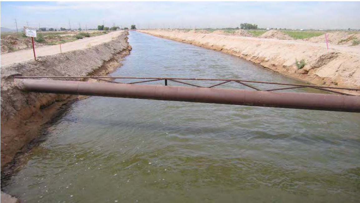
Photo 6. View of the Buckeye Canal and the surrounding land in the project area from Cotton Lane south of MC 85, facing west.
