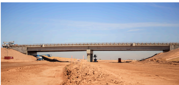
Elliot Road passing over the Loop 202 freeway
