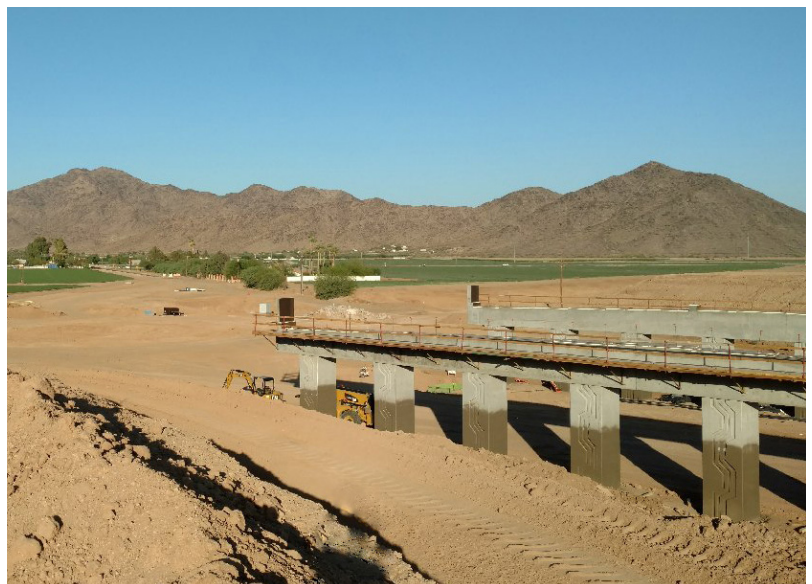
Preparing for girders to be set for the Estrella Drive interchange
