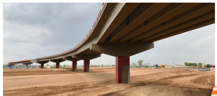
Loop 202 north to I-10 west flyover bridge
