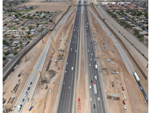
I-10 Papago Freeway access roads between 51st and 67th avenues
