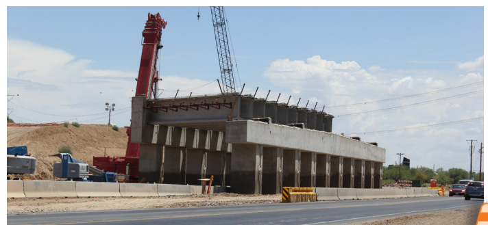
Girders being set on the 51st Avenue bridge
