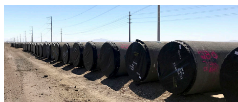
Delivery of the Liberty Lane 48-inch waterline (Photo courtesy of ADOT)
