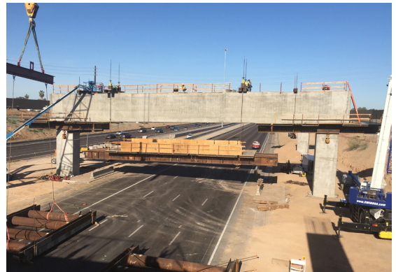
Lowering falsework on bridge west of 59th Avenue
