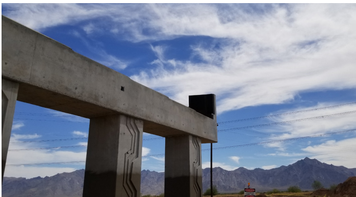
Estrella Drive bridge structure
