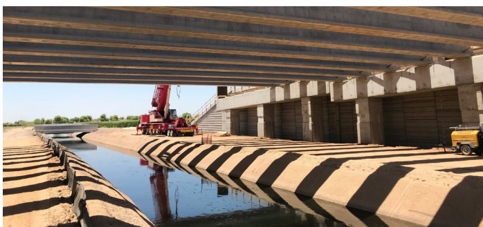
Bridge at the Roosevelt Irrigation District canal
