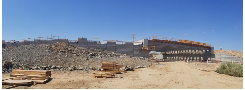
Bridge construction over 24th Street
