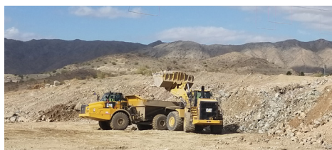
Earthwork near Desert Foothills Parkway
