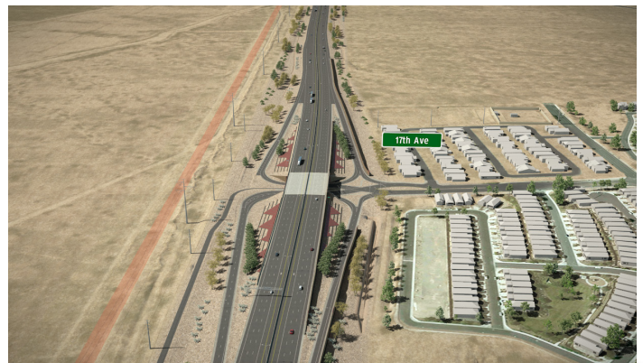
Simulation of the half Diverging Diamond Interchange at 17th Avenue (Image courtesy of ADOT)
