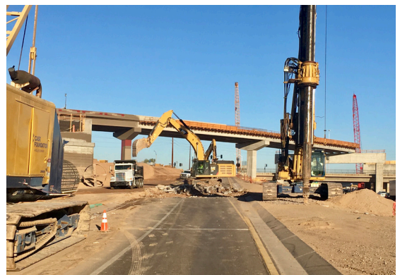
Removal of I-10 eastbound on-ramp at 59th Avenue
