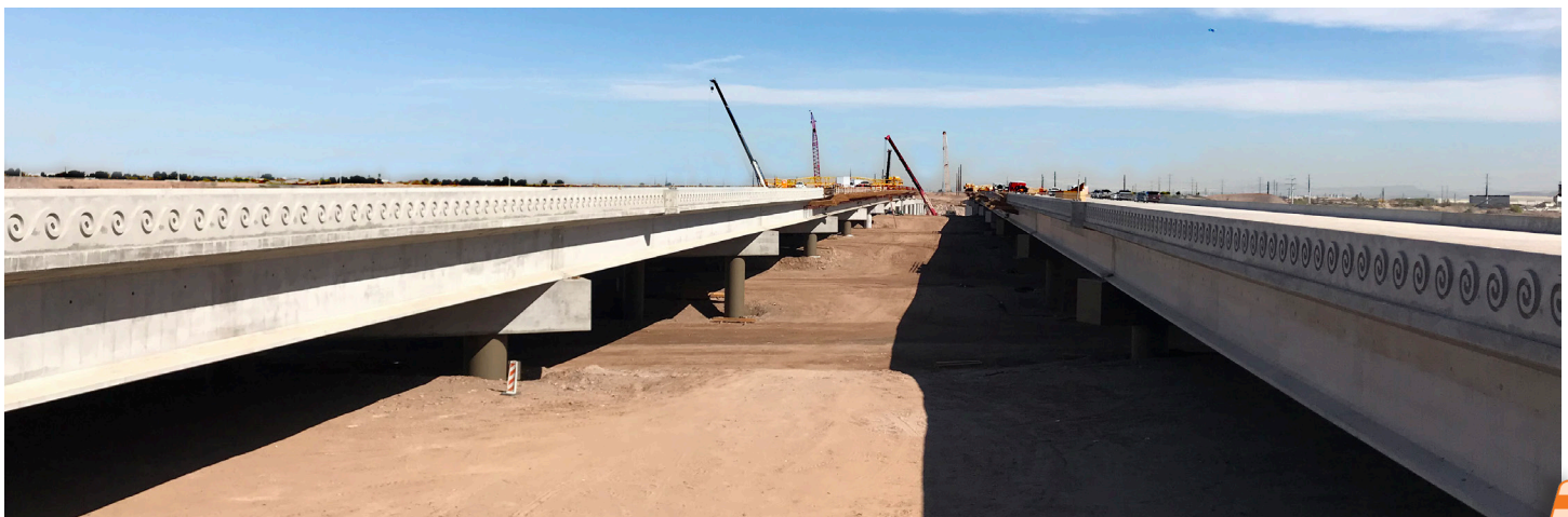
Salt River bridges
