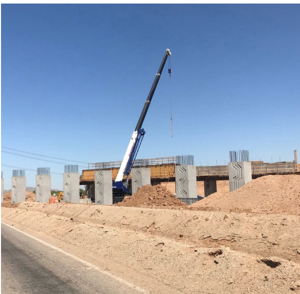
Forming caps for the bridge at Estrella Drive interchange
