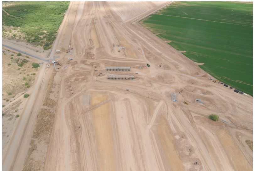
Aerial view of double-roundabout construction at Estrella Drive
