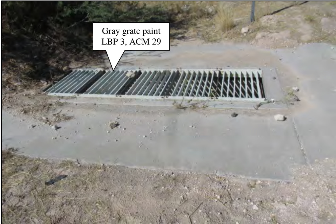
Photograph 7. Detail view West Kingman TI OP WB off-ramp catch basin. Photograph date: October 1, 2019.
