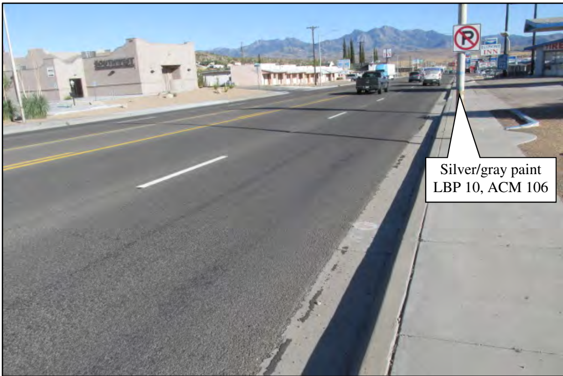
Photograph 28. View southwest of US 93, near MP 70.3. Photograph date: October 1, 2019.
