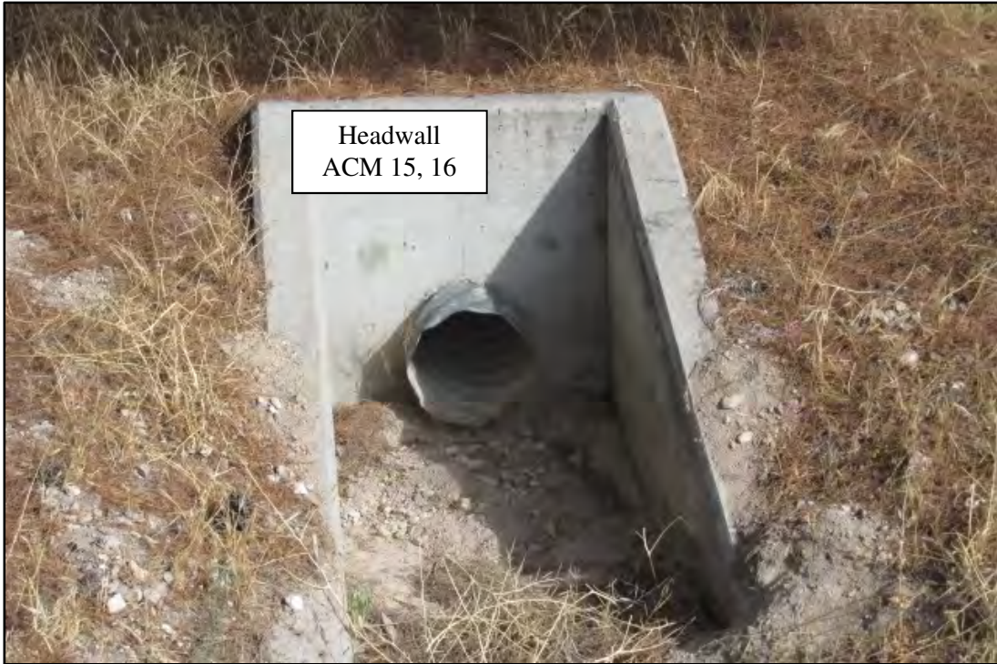
Photograph 9. Detail view of the RCMP at the SWC of the WB West Kingman TI OP. Photograph date: October 16, 2019.
