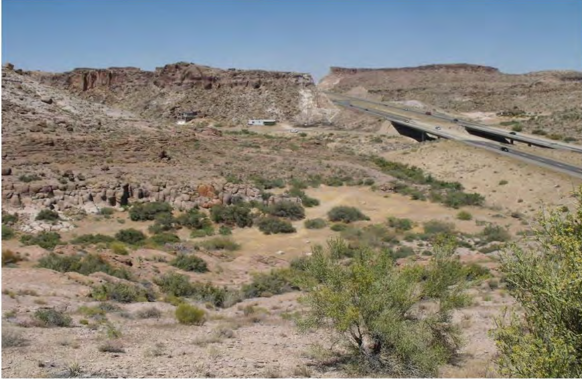
Photograph 3. View to the east of the route for Alternative J3 (June 21, 2012)
