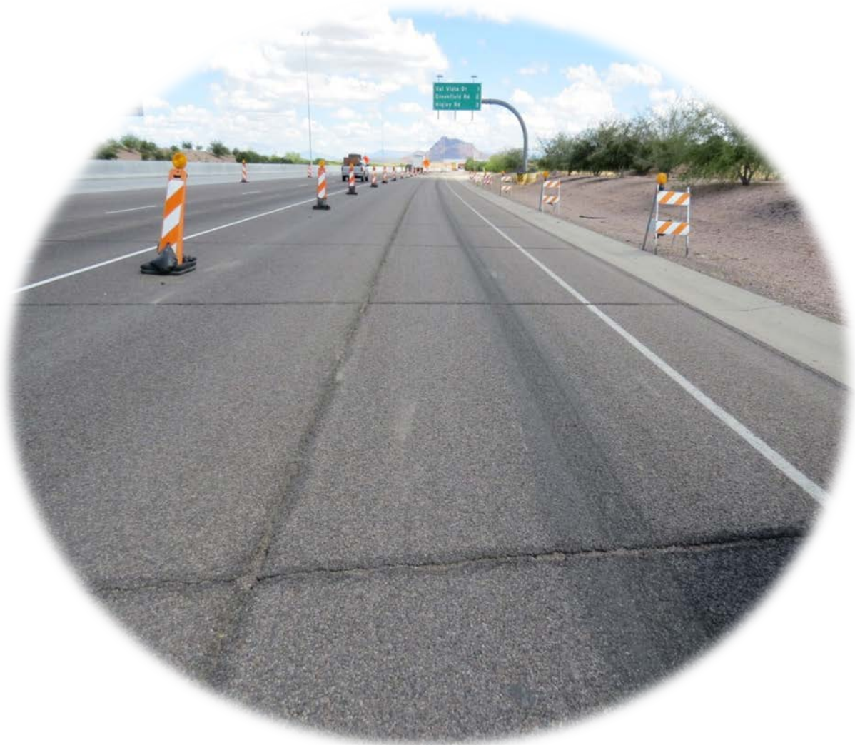
Cracking (Unacceptable)
