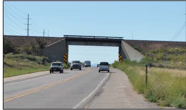
Figure 7 – BNSF Railway Overpass
