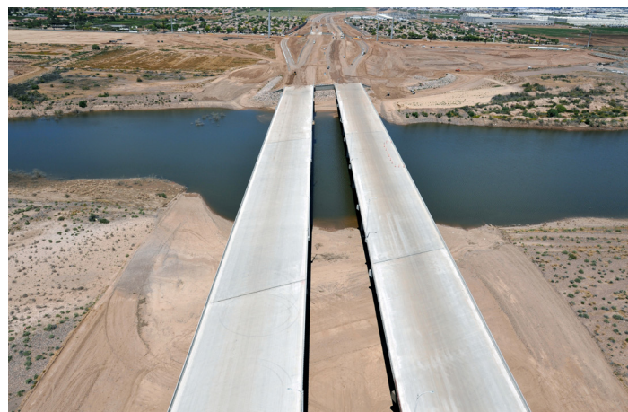
AFTER: Looking north at the bridges over the Salt River April 2019
