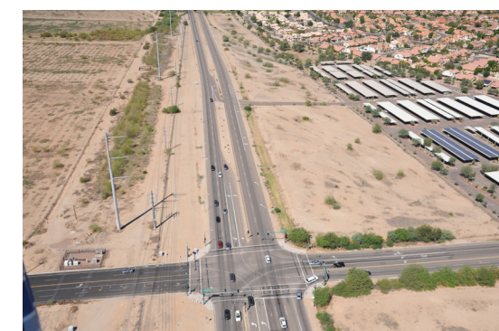
BEFORE: Looking west toward Pecos Road and 40th Street intersection September 2016
