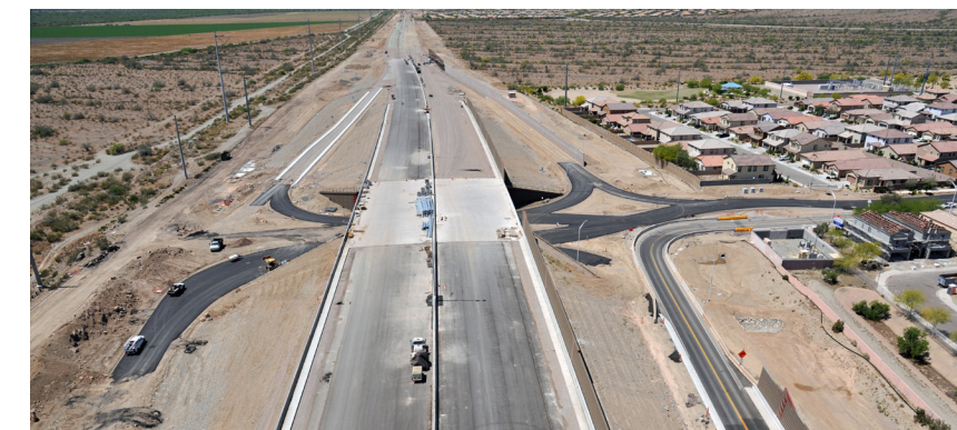
Looking west toward 17th Avenue Diverging Diamond Interchange construction April 2019
