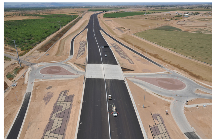
AFTER: Looking northwest toward the Estrella Drive interchange April 2019
