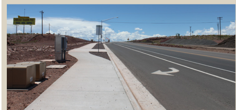
ADOT constructed sidewalks to accommodate pedestrians along US 89 near Cameron.
