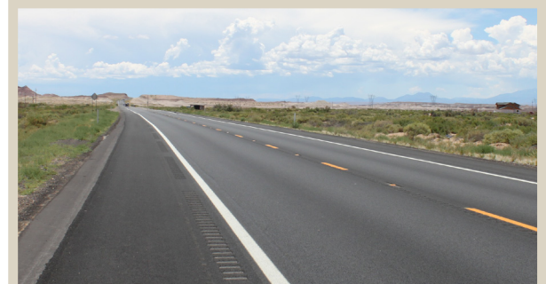
On US 89 north of Cameron, a wide paved shoulder accommodates bicycles and pedestrians.
