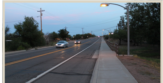
Striped paved shoulder
