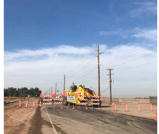
Closing Southern Avenue to expedite construction of street improvements
