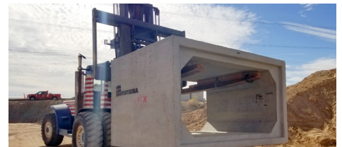
Placing a pre-cast culvert near 24th Street
