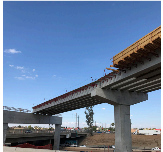
Constructing a flyover ramp from northbound Loop 202 to westbound I-10
