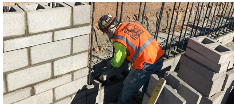
Stacking block for the sound wall near 48th Street
