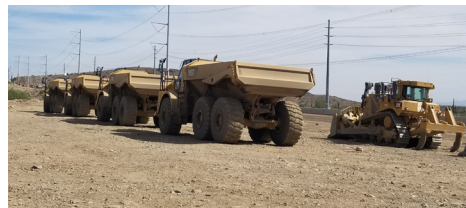
Transporting rock from controlled rock blasts
