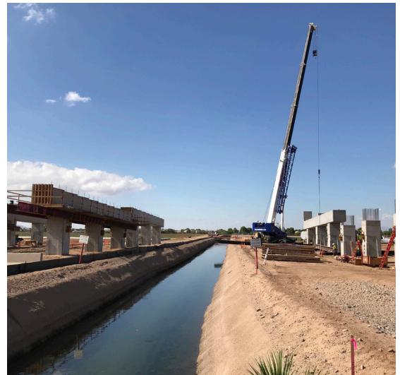
Building piers for a bridge over the Roosevelt Irrigation District canal
