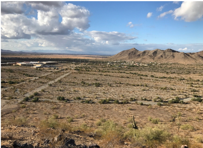
The Center Segment includes approximately three miles of new freeway.
