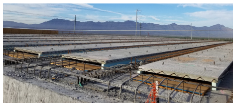
Completing the deck panels on the 17th Avenue bridge
