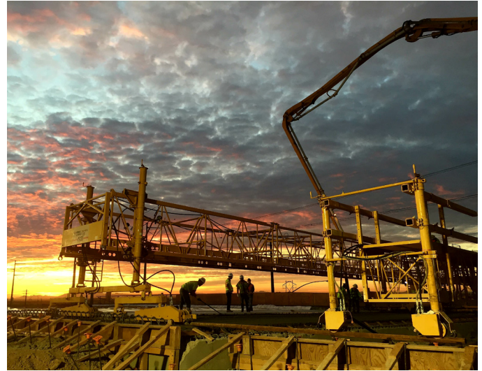
Pouring the 40th Street bridge deck
