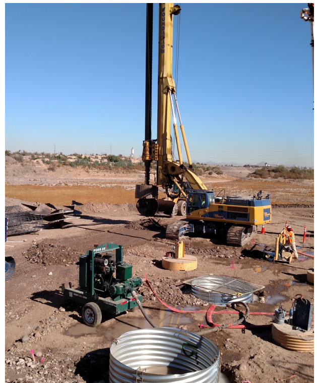
Drilling shafts for bridge piers in the Salt River
