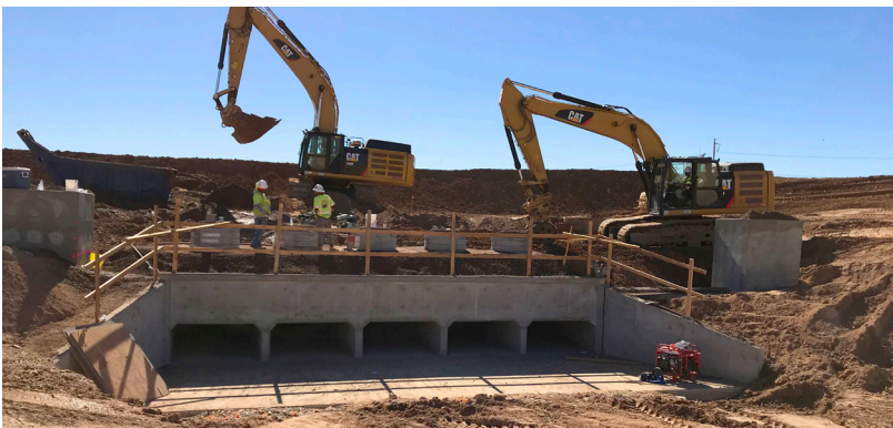
Installing new drainage culvert at Elliot Road
