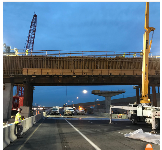
Forming the falsework for a straddle bent over I-10 Papago Freeway
