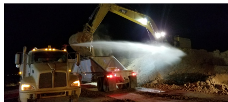
Hauling dirt at night to build the freeway embankment
