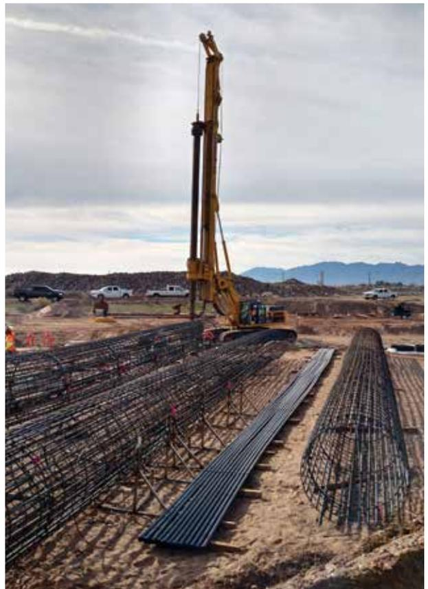
Drilling shafts and installing rebar (ADOT Photo)
