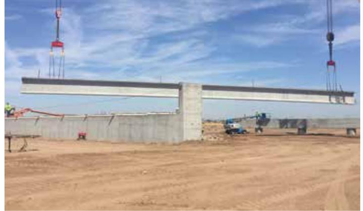
Placing a 174-foot girder, the longest precast concrete girder in Arizona
