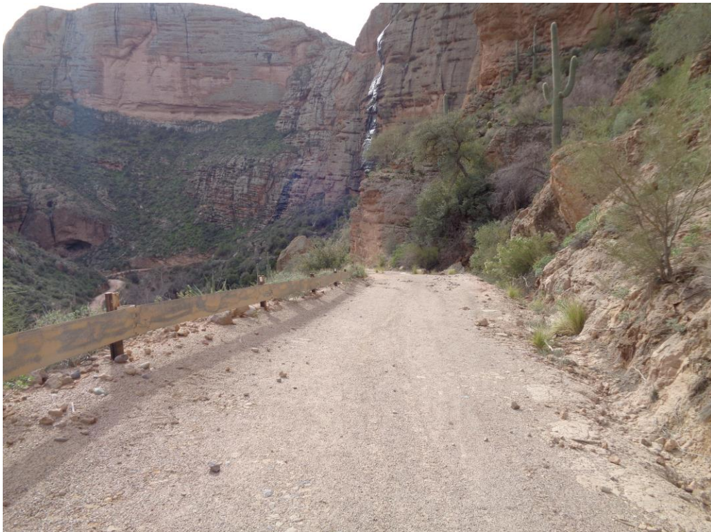
Photograph 10. View of the painted guardrail along SR 88 on Fish Creek Hill.
