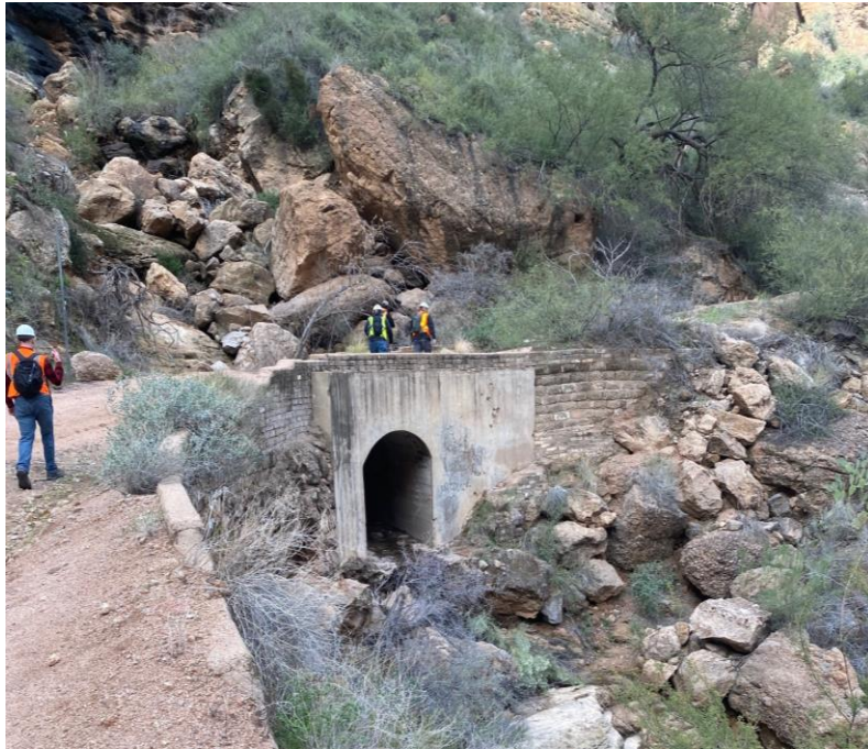
Photograph 13. One of the many concrete structures observed.
