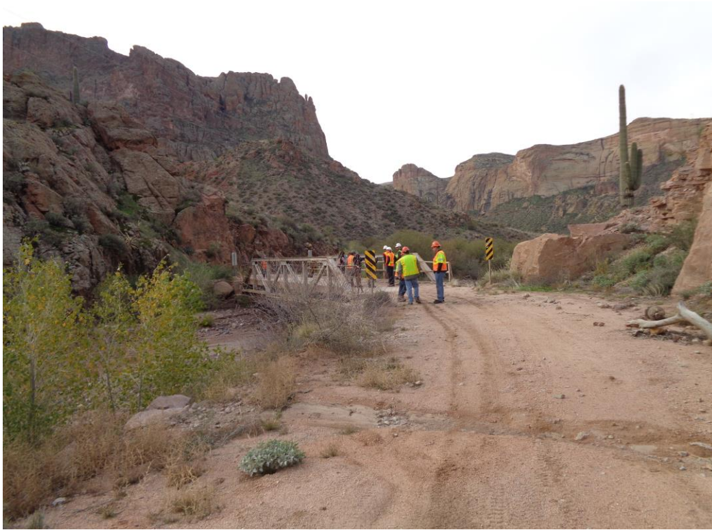
Photograph 1. Overview of the Lewis and Pranty Creek bridge at MP 224.60.
