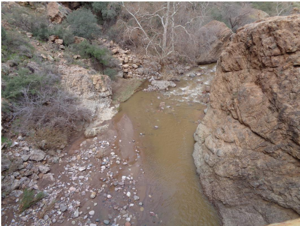
Photograph 6. View downstream at the Fish Creek bridge.
